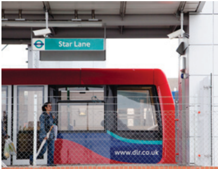
New station open as part of the DLR extension at Star Lane
