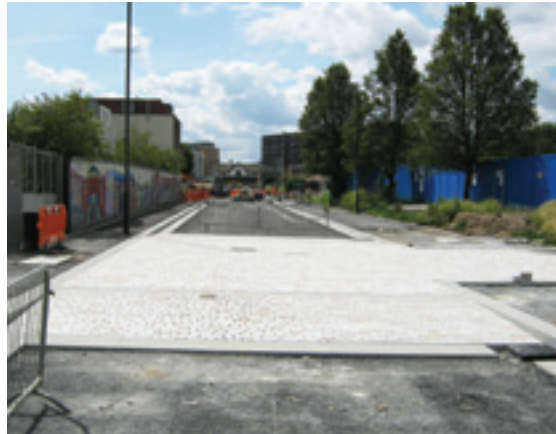
Highways works on Rathbone Street
